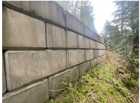
Well founded wall
