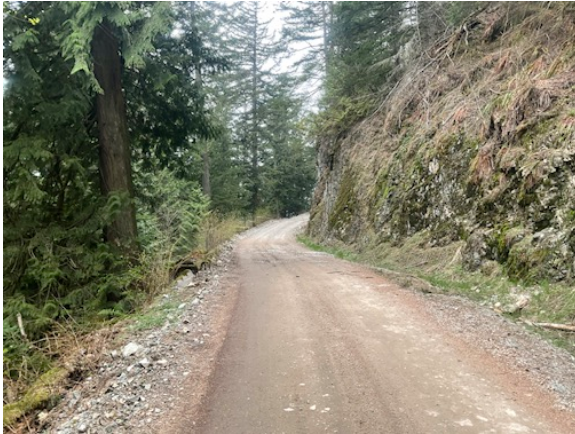
Town approach, ditch needs work.
