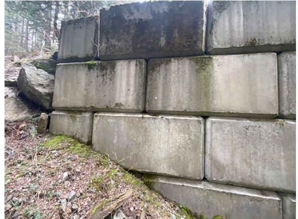
Woods lateral slope. Rip rap with Geo fabric
